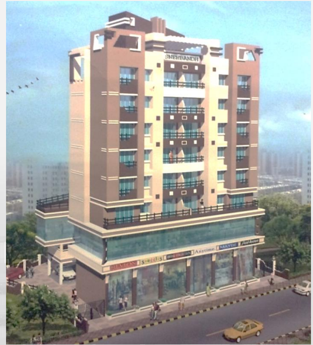
Project Name : Snehbandh C.H.S. Ltd. Location : Yashodhan Nagar, Thane (W) Approx. Cost : 1.75 Cr. Completion Year : 2010 Construction Area : 22,454 sq. ft.
