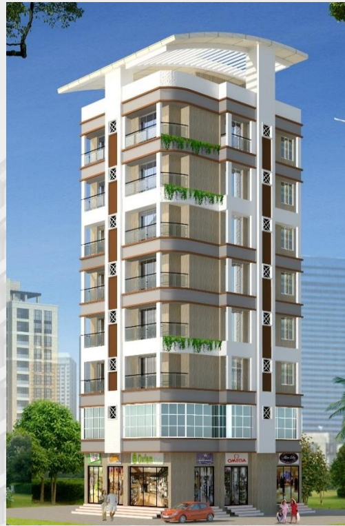
Project Name : Everest Excellence Location : Chendani, Thane (W) Plot Area : 218.20 Sq.Mt. Approx. Cost : 1.05 Cr. Construction Area : 9,900 sq. ft.
