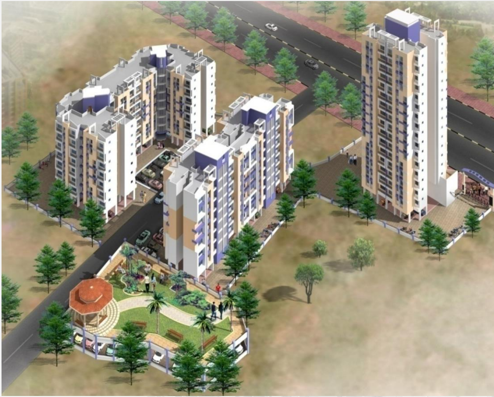
Project Name : Periwinkle Complex Location : Mogharpada , Thane (w) Approx. Cost : 25.41 Cr.
