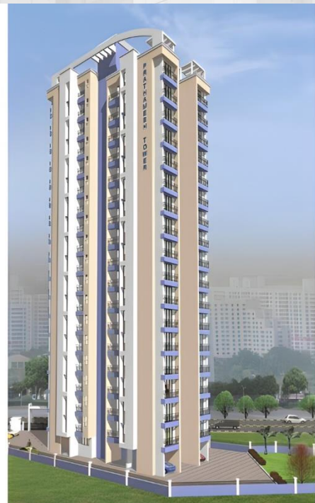
Project Name : Prathamesh Tower Location : Boriwade , Thane (W) Approx. Cost : 10.86 Cr. Completion Year : 2012 Construction Area : 89,559 sq. ft.
